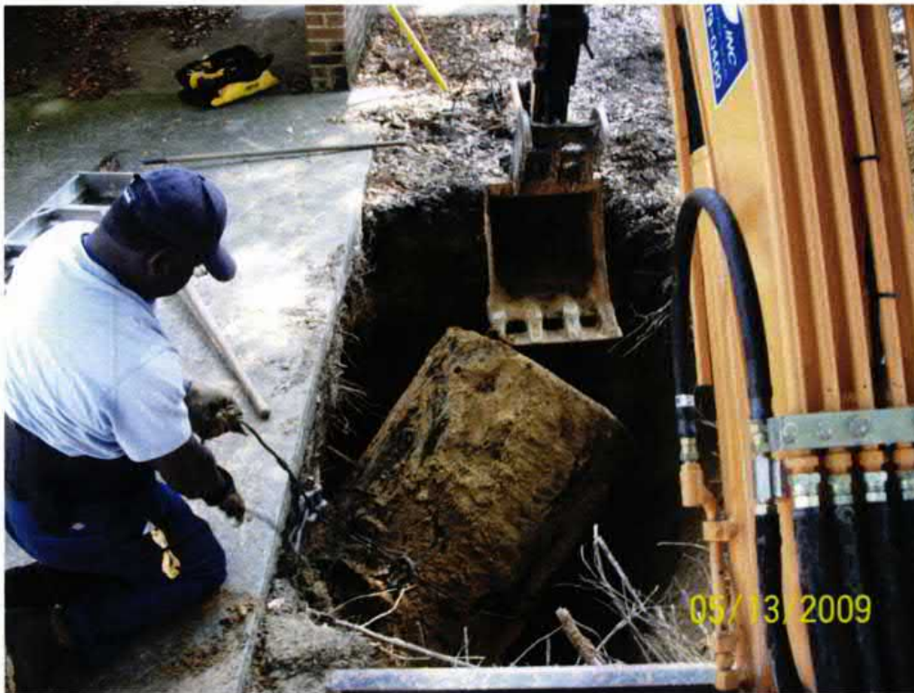
Picture 1: UST 1014Foxglove during removal from the excavation.
